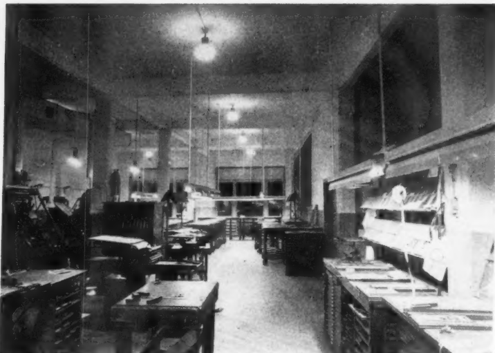
This view of one section of the composing room of the Leader Press, Inc., Oklahoma City printing plant, shows the use of fluorescent lamps in troughs directly above the composition tables at the right in the photograph and in the back of the room. General illumination is provided by conventional incandescent units at the ceiling.
